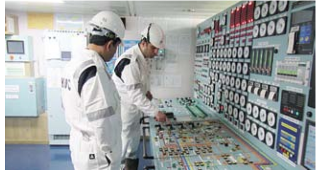
■ Inside the cargo control room
